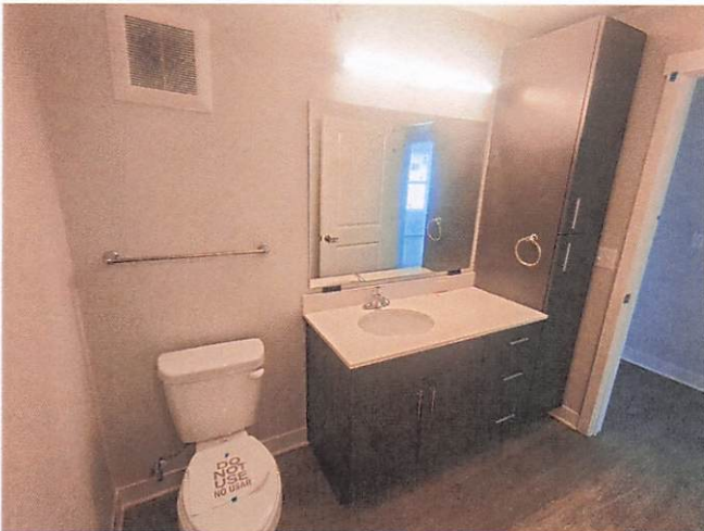
Bathroom finishes Building A
