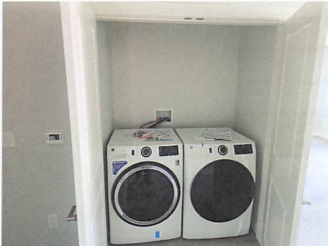
Appliance installation in building A Level 3
