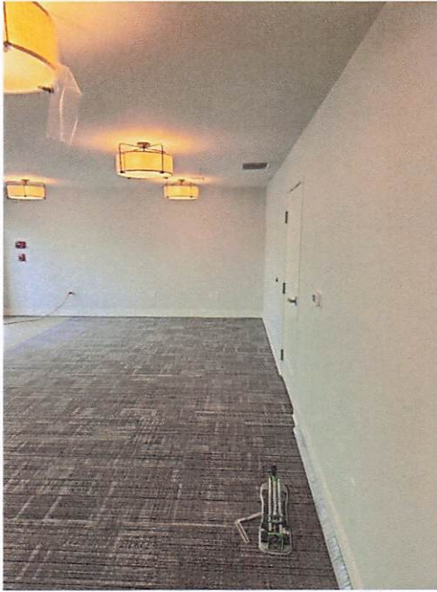
Building A finishes continued
