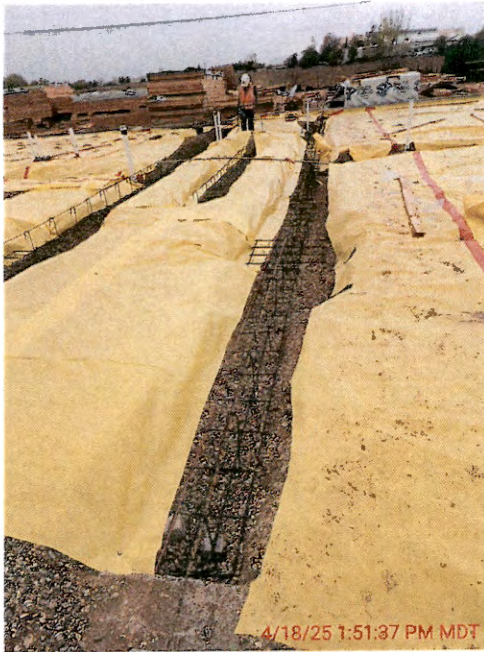
Footings and vapor barrier installation
