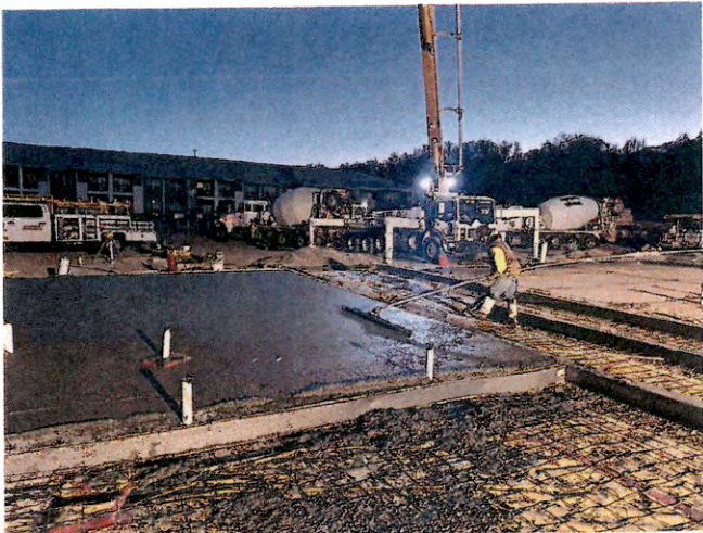
Concrete slab on grade installation Building A
