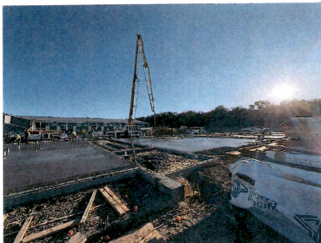
Concrete slab pouring building B
