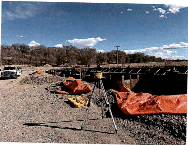
Surveying Building A for concrete pour
