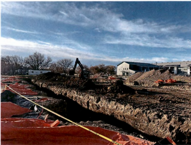
Excavation of buildings footings
