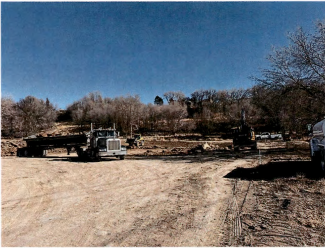
Site grading and earthwork.
