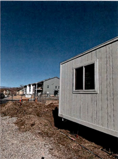
Construction trailer arrives on site
