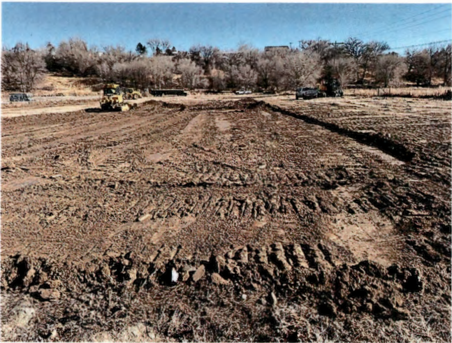
Initial earthwork, and site fence installation
