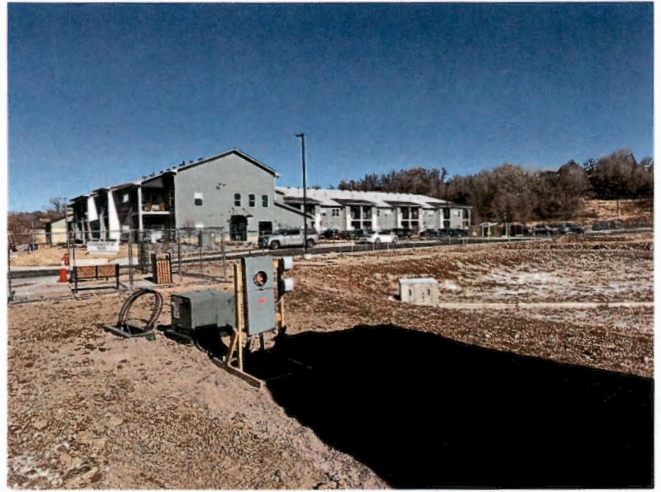
Electrical temp power installed
